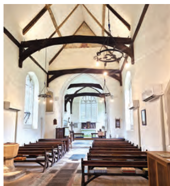
Air to air heat pump heaters
