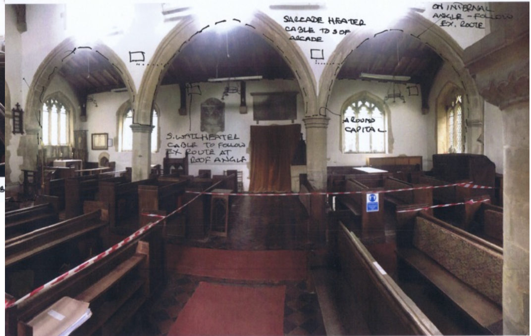
PETERS UPWOOD S. ARCADE / S. WALL HEATERS & CABLE ROUTES
